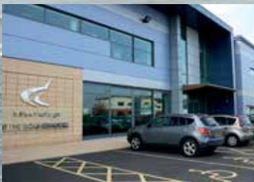
Roundhouse Johnson Building
